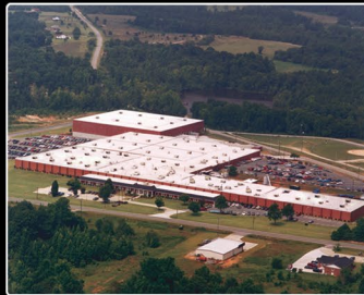
PAGELAND, SC Final Assembly and Distribution Center
