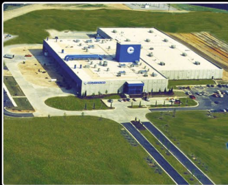
PAGELAND, SC Bronze Foundry and Manufacturing Plant
