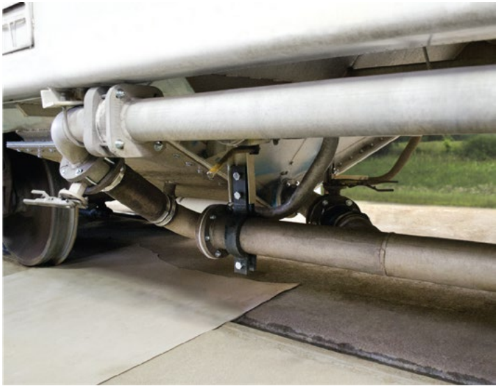
Photo courtesy of Economy Coating Systems, Inc.® - Camanche, IA
